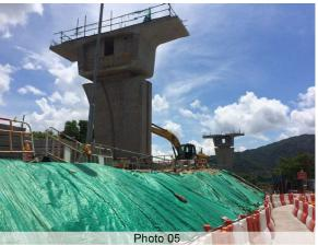
Hydroseeding on soil slopes and sheeting of soil stockpiles to prevent erosion and dust generation with visually unobtrusive material
