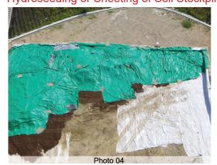
Sheeting of soil stockpiles to prevent erosion and dust generation with visually unobtrusive material
