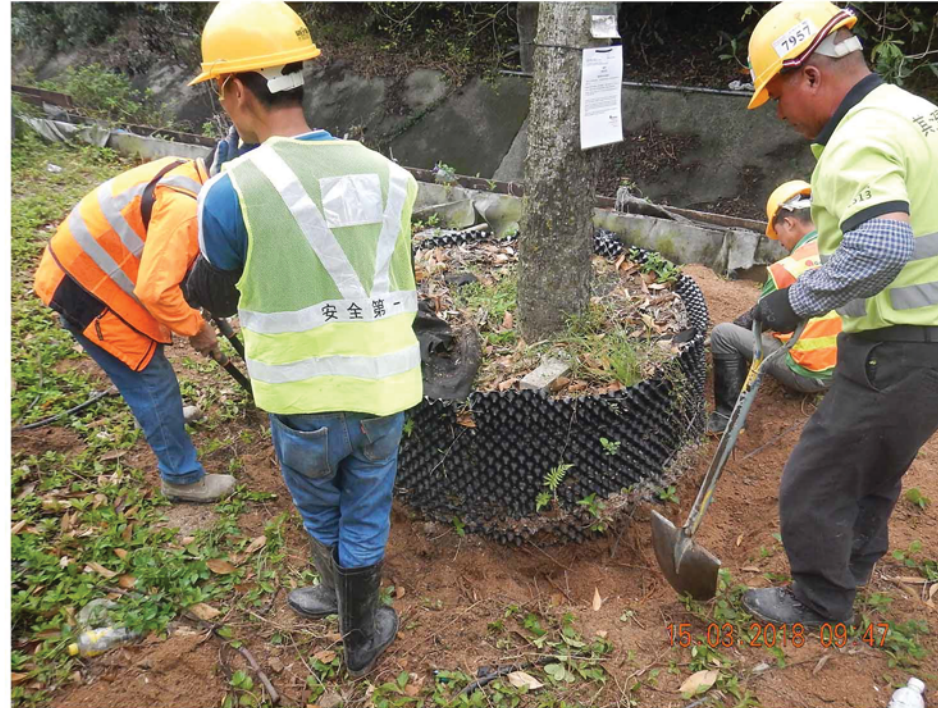
PREPARATION OF ROOTBALL
