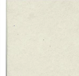
Roof Floor Tiles
