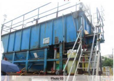
Site runoff was collected and treated in the waste water treatment facilities before discharged into the adjacent water bodies.
