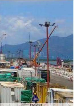
Lighting in the Southern Landfall is subject to the requirement on aviation aspects. Lights shall not form a source of glare or in any way affect pilots and air traffic controllers.
