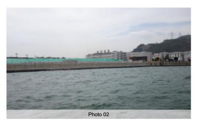
Sheeting of soil stockpiles to prevent erosion and dust generation with visually unobtrusive material
