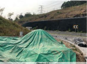
Hydroseeding on soil slopes and sheeting of soil stockpiles to prevent erosion and dust generation with visually unobtrusive material.
