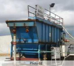
Site runoff was collected and treated in the waste water treatment facilities before discharged into the adjacent water bodies.
