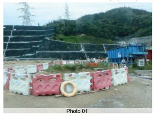
Site runoff was collected and treated in the waste water treatment facilities before discharged into the adjacent water bodies.
