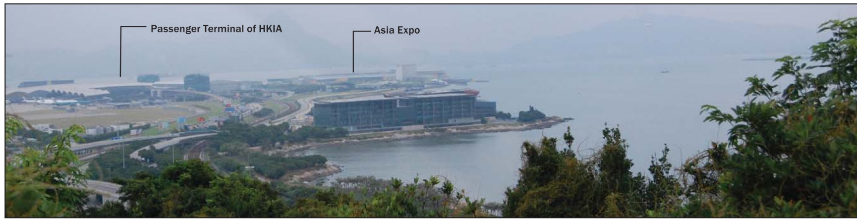
Existing Baseline Condition - Viewing Towards HKBCF (Day 1 of Construction Phase)
