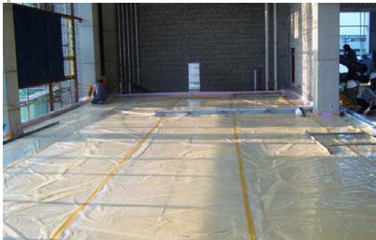
Spread 2 layers of vinyl sheet in the PO-MAT
