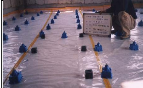
Sep-up Jack-up mount on vinyl sheet after cleaning
