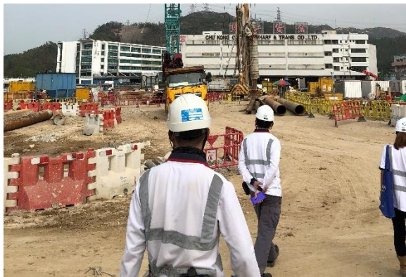
Photo 3 - Unpaved roads were maintained in a wet condition (12 October 2018)
