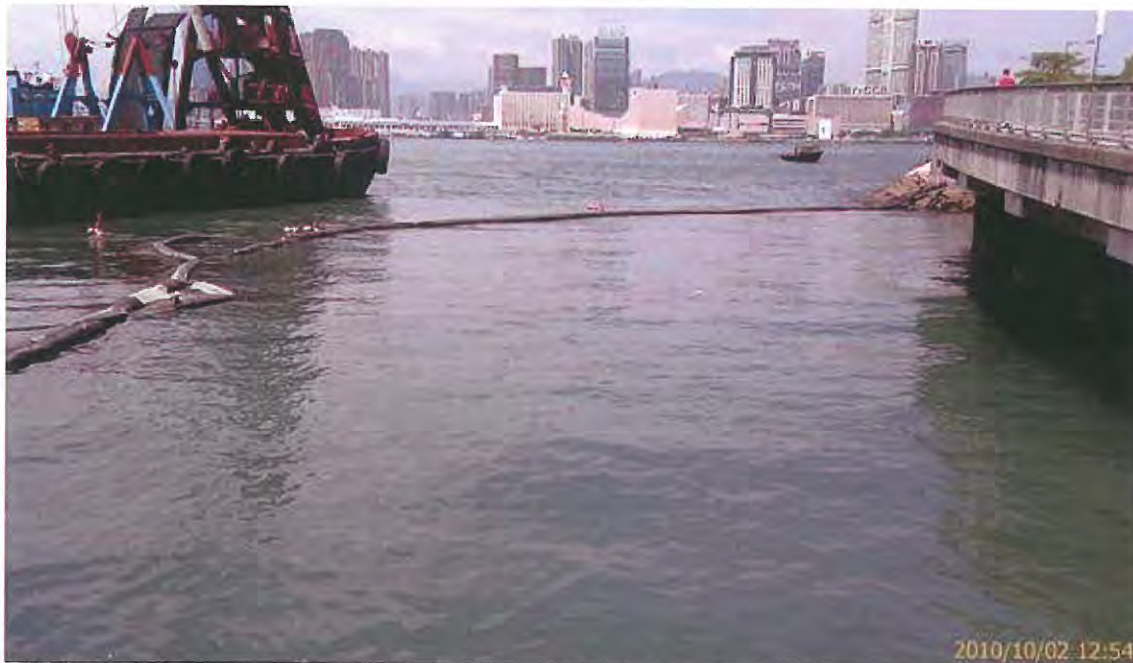
SG110/110 woven geotextile use as silt protector at Wanchai Development Phase II, Oct 2010
