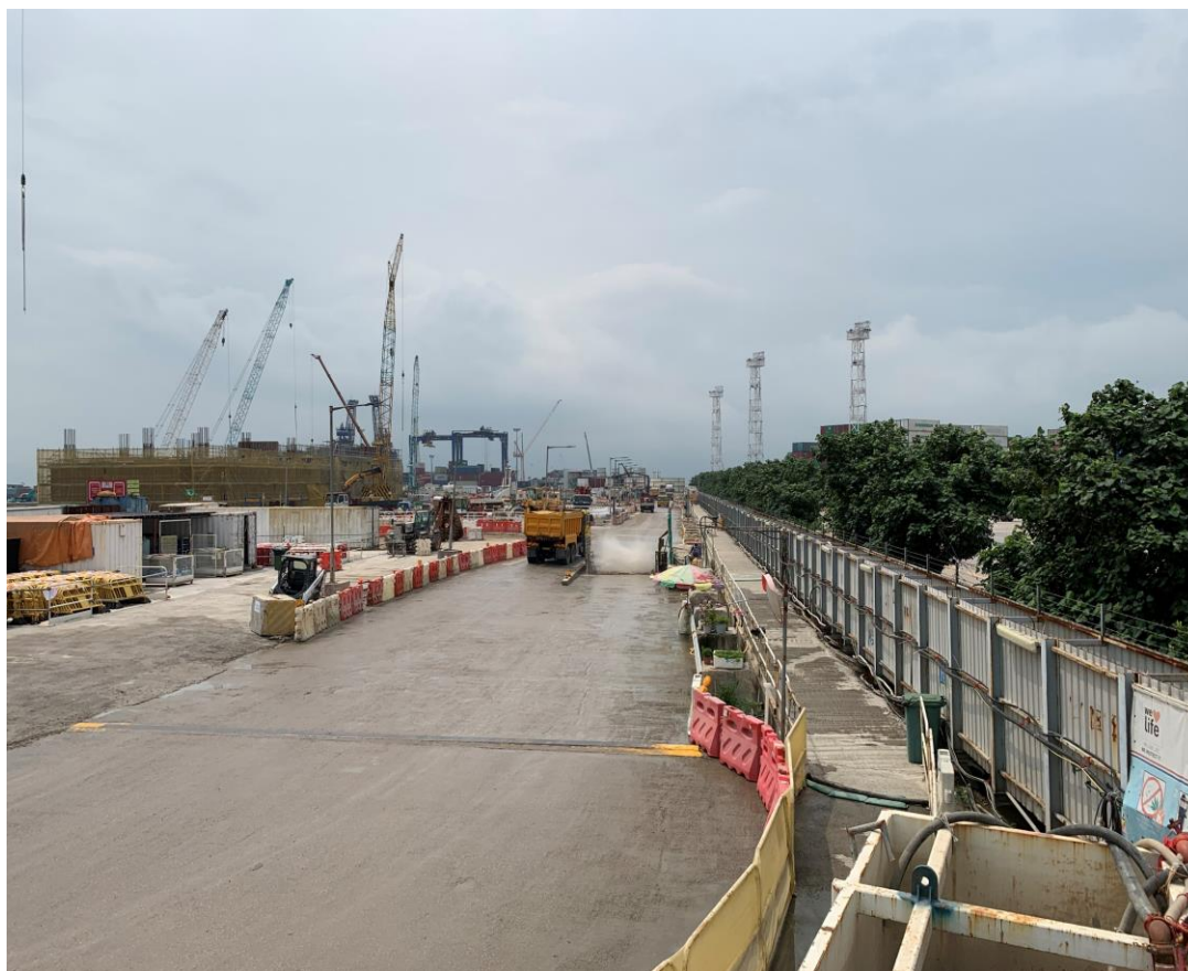
Water spraying was applied at the main haul road to prevent dust. (Works Area Portion N-A)
