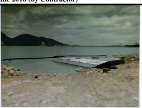
2. 16 June 2018: Silt curtain at Box Culvert C was observed as secured. No leakage of muddy water into the open waters was observed.
