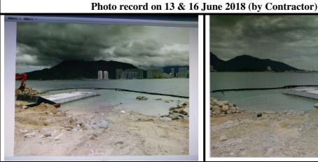
1. 13 June 2018 (daytime): Silt curtain at Box Culvert C was observed as secured. No leakage of muddy water into the open waters was observed.
