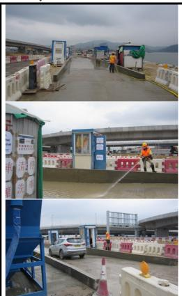
2. Water spray implemented at HY/2013/04 site boundary for vehicles leaving HY/2013/04 site towards BCF Island site exit. No specific observation referring to air or water quality mitigation measures associated with the wheel wash facility was observed.
