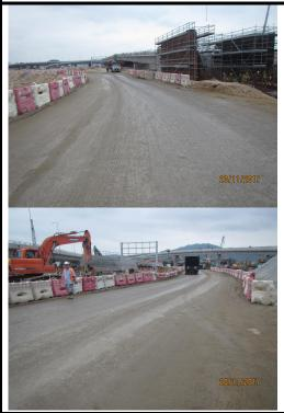
1a. Water spray provided for haul roads in the HY/2013/04 site area (near Box Culvert C). No fugitive dust generation was observed.
