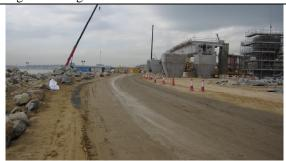
1c. Water spray provided for haul roads in the HY/2013/04 site area (near Bridge D12). No fugitive dust generation was observed.
