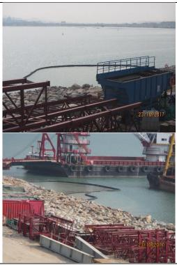
3. Silt curtains provided for marine work areas at Box Culverts  $\boldsymbol{C}$  and  $\boldsymbol{D}$ .
