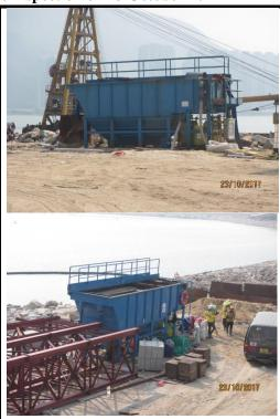
2. Wetsep provided near Box Culverts C and D to treat site runoff before discharge from the contract site. No discharge was observed at the discharge points or along the same shoreline interfacing with open waters.
