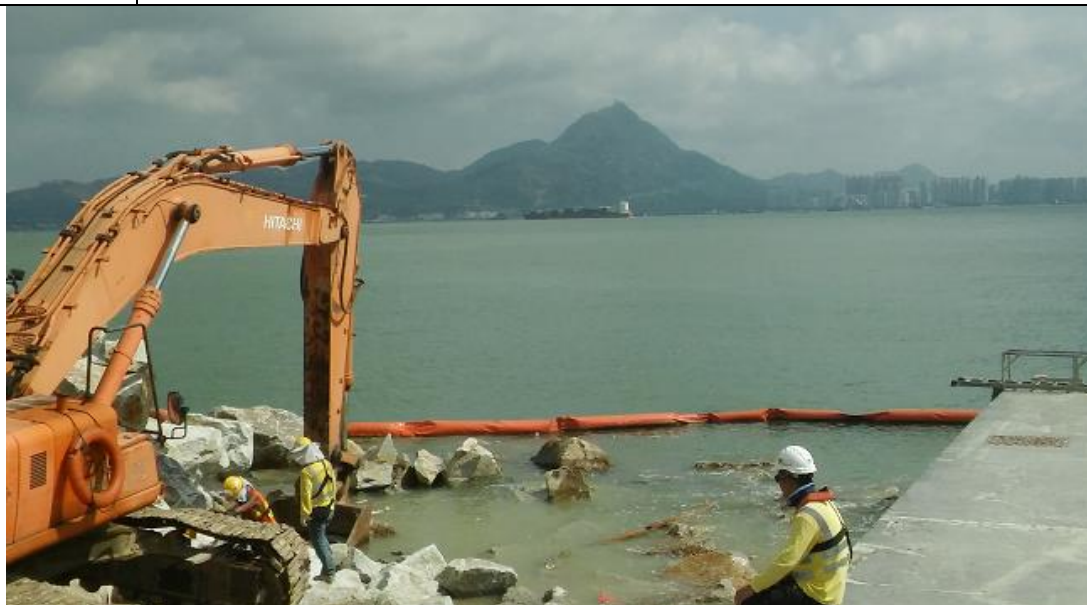
Photo 3 | Construction of seawall
