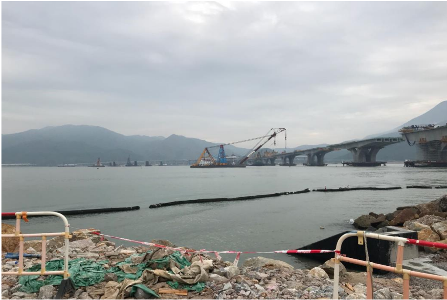
Photo record show silt curtain condition and active seawall construction area on 8 Nov 2017.
