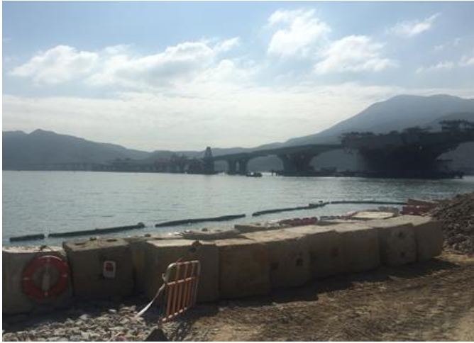
Photo record show silt curtain condition and active seawall construction area on 9 Nov 2017.
